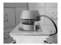
2.) Note the location of the wires. Disconnect and remove the wires from the junction box.
